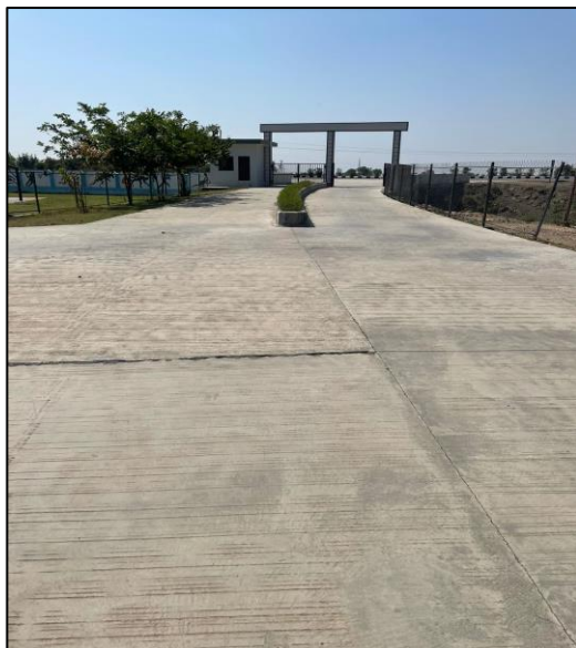
Figure 13 - Concrete Road within the college premises
