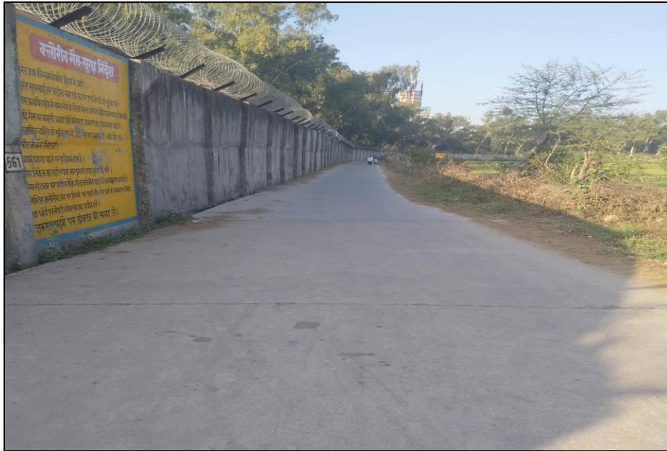
Figure 16 - Construction of cement concrete towards Gadepan from Pachra, Kota
