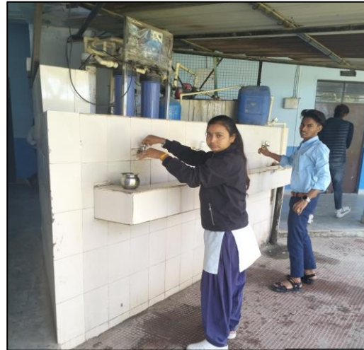
Figure 12- Drinking facility at ITI Baran
